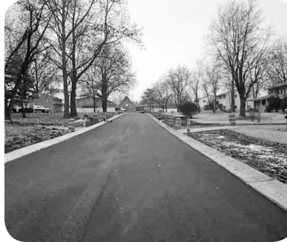
Vero Lane Under Construction
