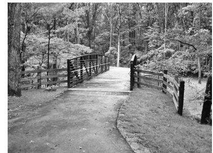
Bluebird Park's Oakhill Trail bridge
